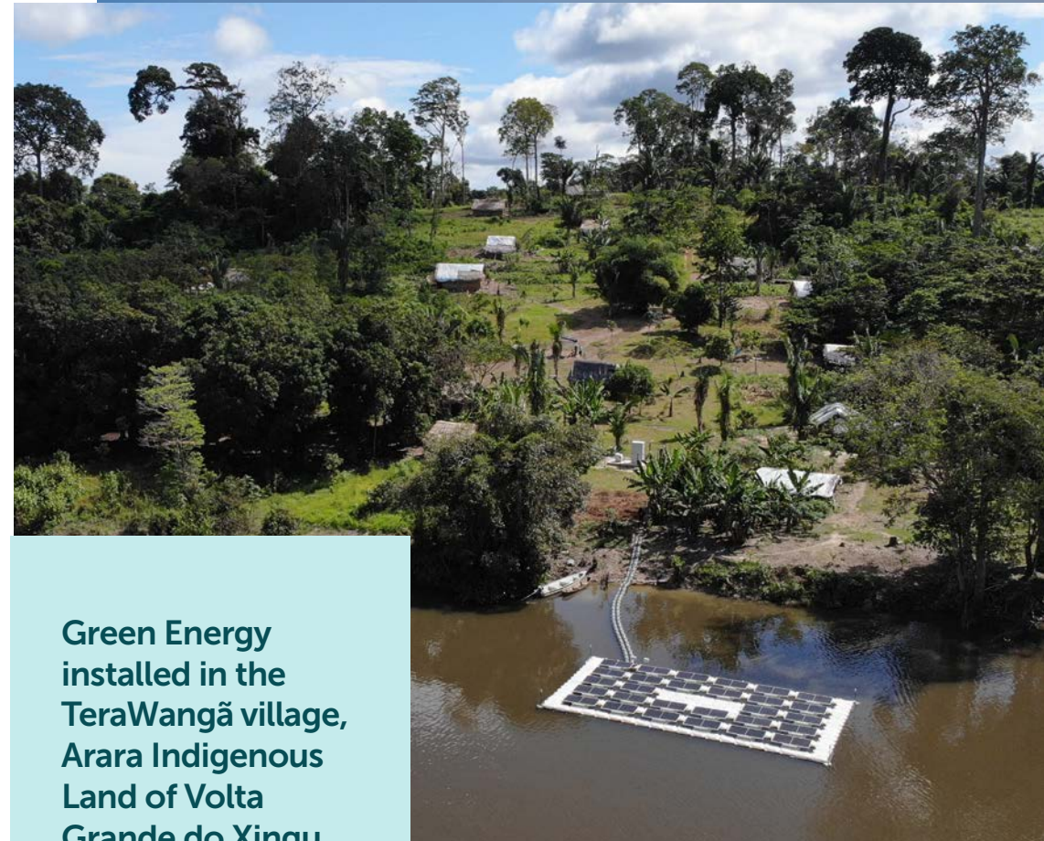
Green Energy installed in the TeraWangã village, Arara Indigenous Land of Volta Grande do Xingu
