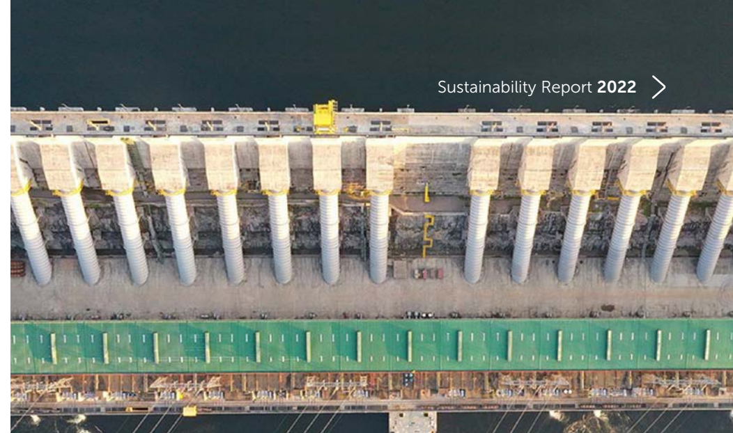
Aerial photo of the Belo Monte HPP Main Powerhouse
