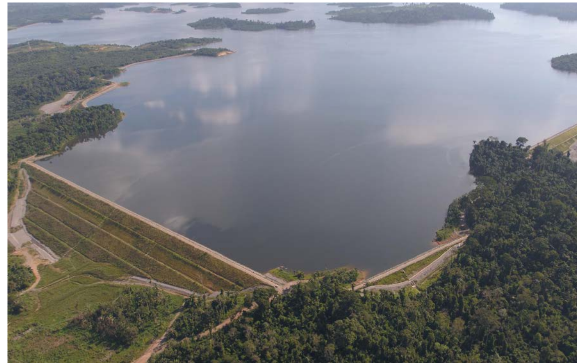
Aerial view of Dyke 14C
